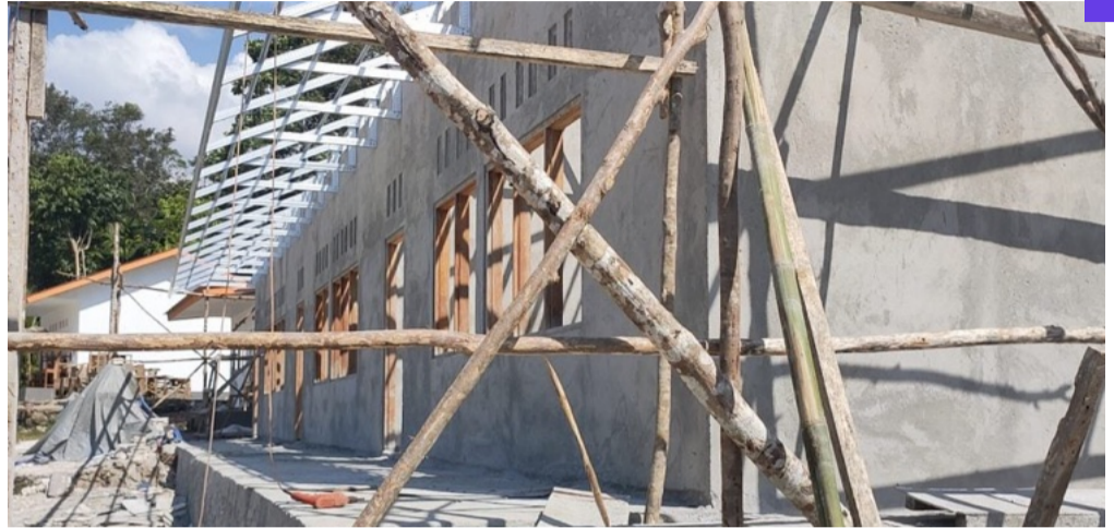
Wali Ate school construction
