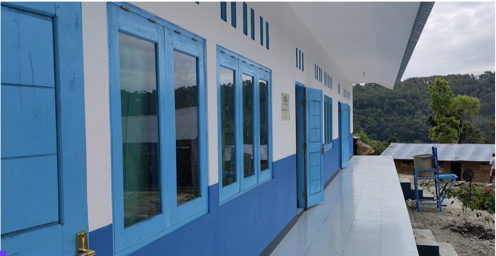
Wali Ate school construction
