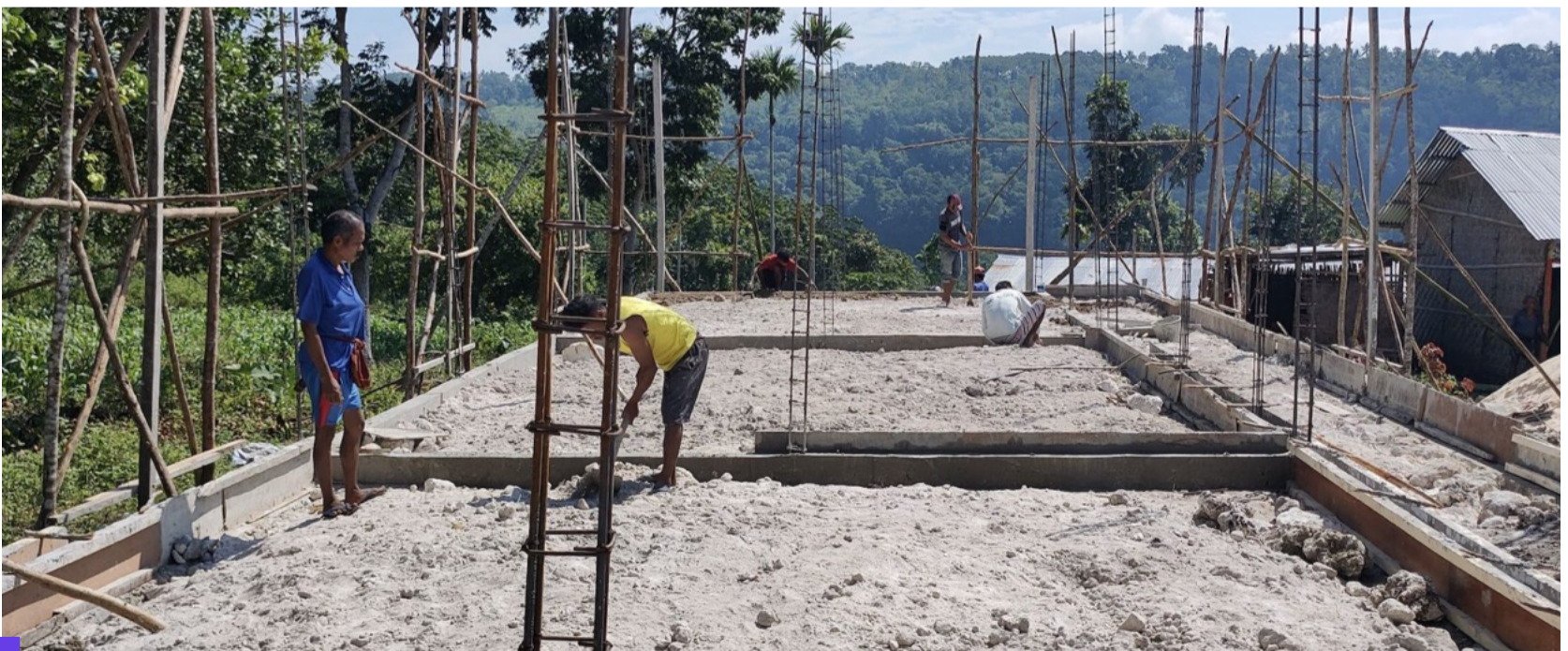
Wali Ate school construction
